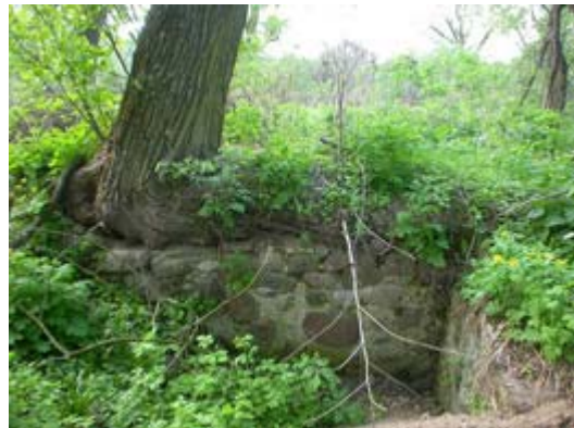
Rests of walls
